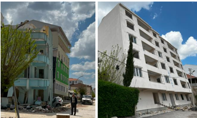
Fig. 5 Buildings leaning on their sides due to the earthquake
