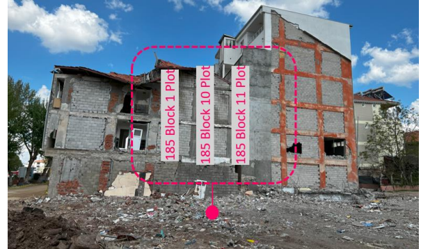
Fig. 3 Collapse of a commercial and residential buildings
