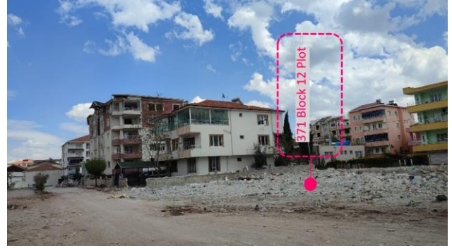
Fig. 2 Collapse of a commercial and residential building
