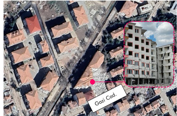
Fig. 6 Damaged building due to design features
